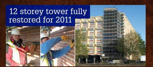
ASRS were asked to investigate and provide a solution to the connecting tower between two residential housing blocks, that had suffered from cracking and movement, as part of planned maintenance by a housing association.
