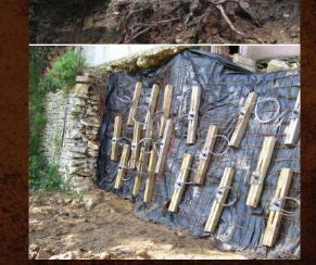
Due to a partial collapse of this retaining wall ASRS were asked to design a permanent solution to stabilise the ground.
