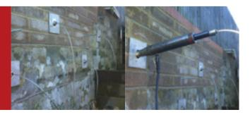
Long Section: We installed 9 No. Platipus S08 lateral restraint anchors with 8mm stainless steel wire tendon, driven to 4m or refusal, terminated onto 200mm dia square load plates with 8mm stainless steel wedge grip set on the face of the wall. In addition we also installed 4 No. twin bands of Helibar 60 stainless steel bed joint reinforcing, positioned horizontally to distribute the structural loads, returned to the right flank section of the wall.
